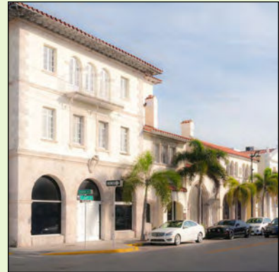
[ taller building anchoring block corner ]
