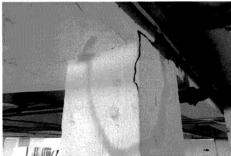
Figure 12 – Concrete spalling at top of supporting column. Repair Type A required.
