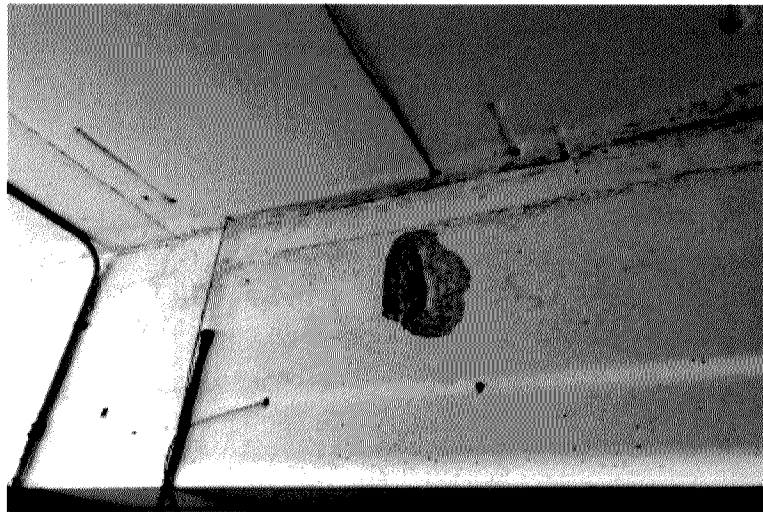
Figure 13 – Exposed reinforcement and concrete spalling on precast beam. Repair Type A required.
