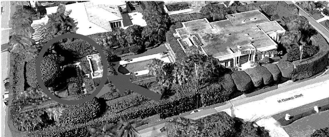
Area of new accessory structure
