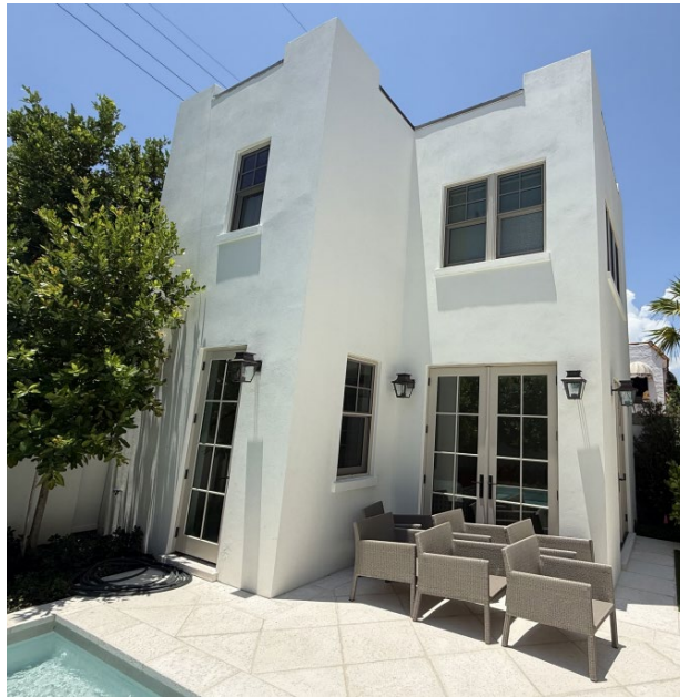
Photograph of accessory structure.
