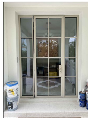
Conditions post inspection (vertical muntins added).
