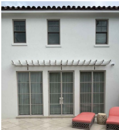
Conditions at inspection.
