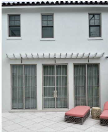
Conditions post inspection (vertical muntins added).
