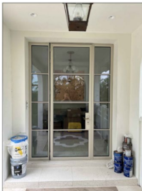
Conditions at inspection.
