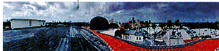
IMAGE 4 - THEATRE ROOF: PANORAMA VIEW OF EXISTING ROOF
